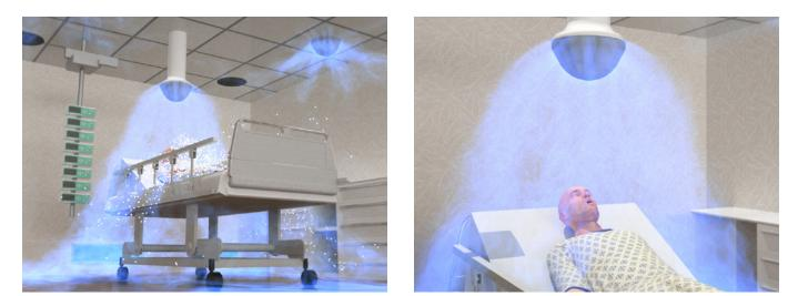
Avidicare ventilation system creates an "air shield" around the head of the patient. It plays two roles: avoiding risk for the medical staff while operating around the head of the patient—particles are moving downward and then extracted; and second, keeping the patient safe from airborne pathogens present in the room.
