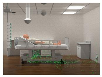
Green particles are potential airborne pathogens coming from outside the room. Thanks to the Avidicare ventilation system, the particles remain near the floor and are extracted directly behind the bed far away from patient to avoid any risk for the patient.
